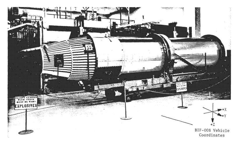
Note: Hardware shown is representative of FM-47. FM-48 differs in that the aft diameter of SRV 1 is slightly greater than the forward diameter of the ejectable adapter.
