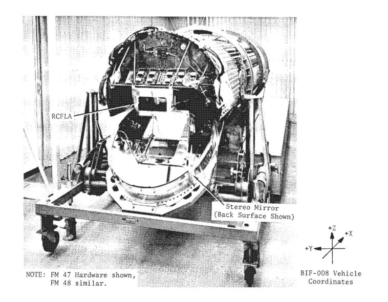
Figure 4.3-4. Assembling Stereo Mirror to COA
