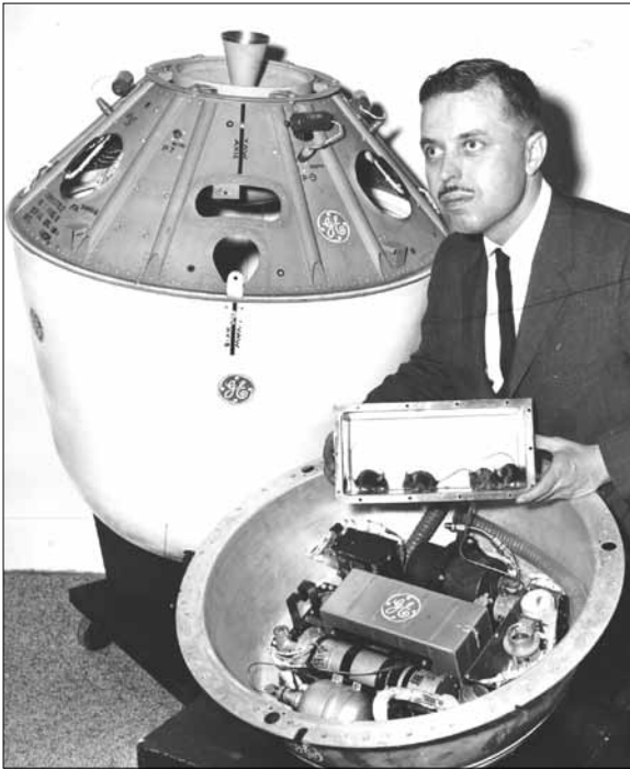
Figure 44. Ingard Clausen, Project Manager of General Electric's (GE's) team, which constructed and instrumented the life capsule, examines four mice, cousins and exact duplicates of those in orbit aboard Discoverer 3. Photo courtesy of GE/U.S. Air Force.
